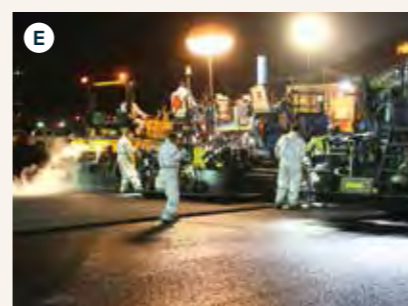
Main runway overlay successfully completed in November.
