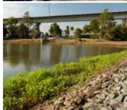
Top: BAC takes advantage of Queensland's sunshine as part of its renewable energy program Bottom: Lake McMillan is an important recycled water catchment for BAC
